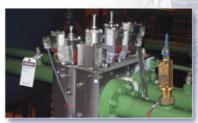
Monitoring the temperature of the hydraulic fluid in a 2/2 way-valve
